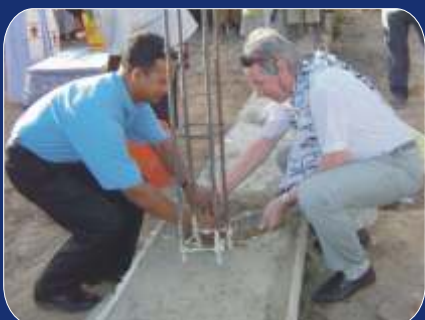
Mr. Werner laying foundation for the Prep School
