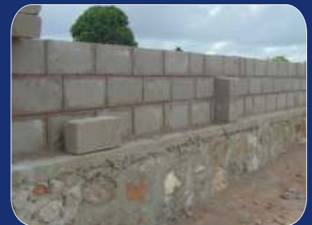
The 2nd Phase of the Primary School Construction progresses
